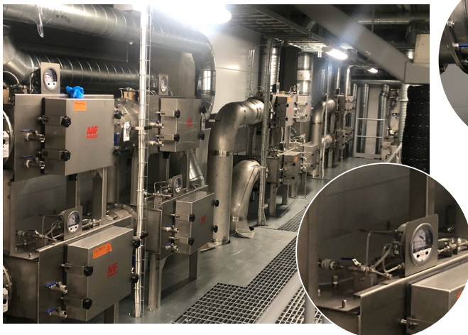
DIN test port for test filter gasket leakage (separated from contents with in-line Hepa) and Aerosol feeding port.
