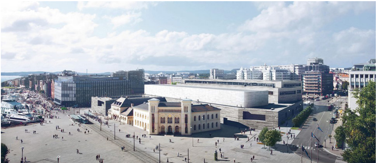
The National Museum of Art, Architecture and Design, Oslo; Planned completion: 2020; www.nasjonalmuseet.no/en/
