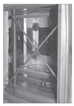
Seismic Cross Bracing
